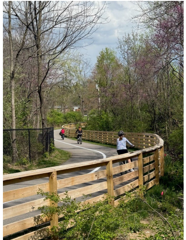
Contractors completed painting a center line along the curved segments of trail near Town Hall on the Big-4 Rail Trail.
