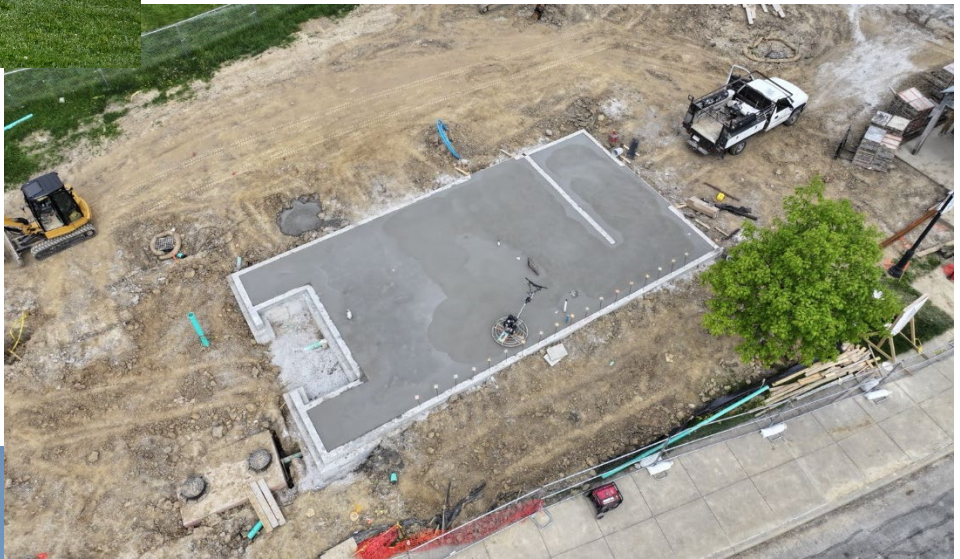
Things are on the rise! The foundation for the Mulberry Fields concession stand is poured and the walls are beginning to go up.
