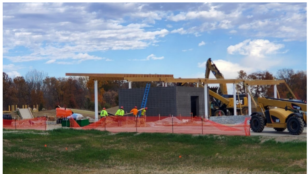
Progress continues at CNP with the Prairie Pavilion going vertical
