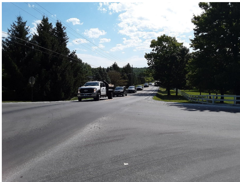
CR 300 South at 975 East Looking East
