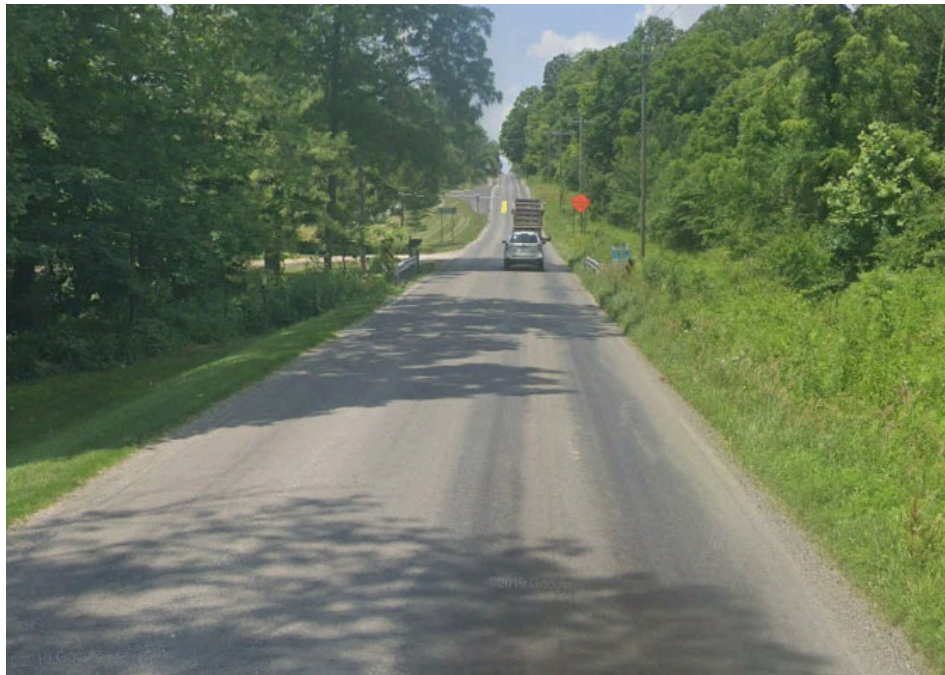
Boone County Bridge 06-00401
