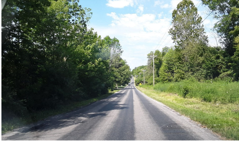
CR 300 South East of Bridge 06-00401 Looking West
