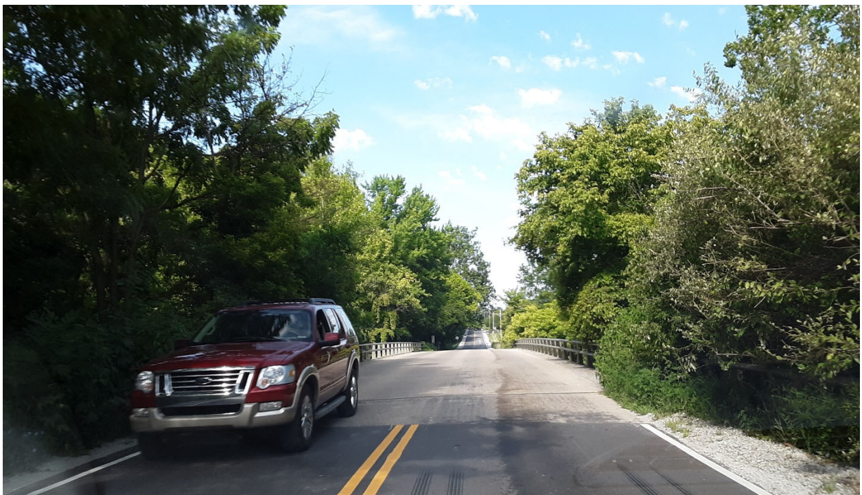
Boone County Bridge 06-00189
