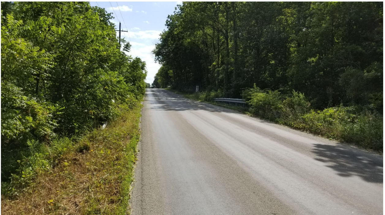
Boone County Bridge 06-00192
