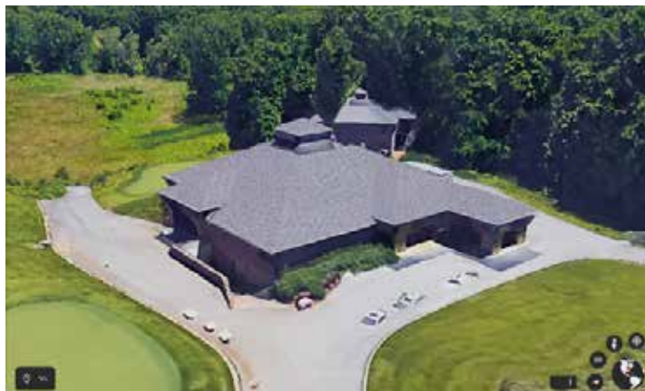
Axon of NW corner of existing Clubhouse
