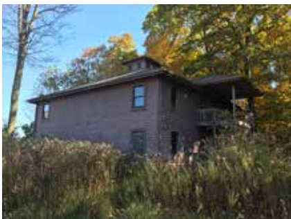
Existing Bunkhouse structure
