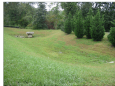
Dry Pond: Photo courtesy of Fairfax County VA Department of Public Works and Environmental Services.
