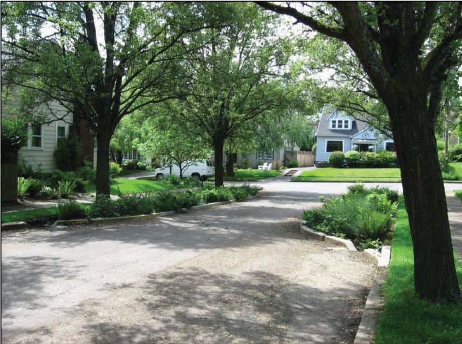
Curb cuts and vegetated areas along a Portland, OR street (USEPA, picasaweb)
