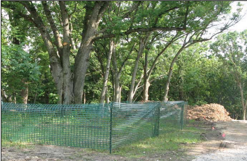
Areas where heavy equipment is not allowed are fenced off to avoid compaction of soils and damages to vegetation (MD Custom Homes, WI)
