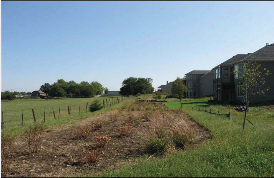
Long swales utilized in areas of natural drainage pathways, Lenexa, KS (USEPA, picasaweb)
