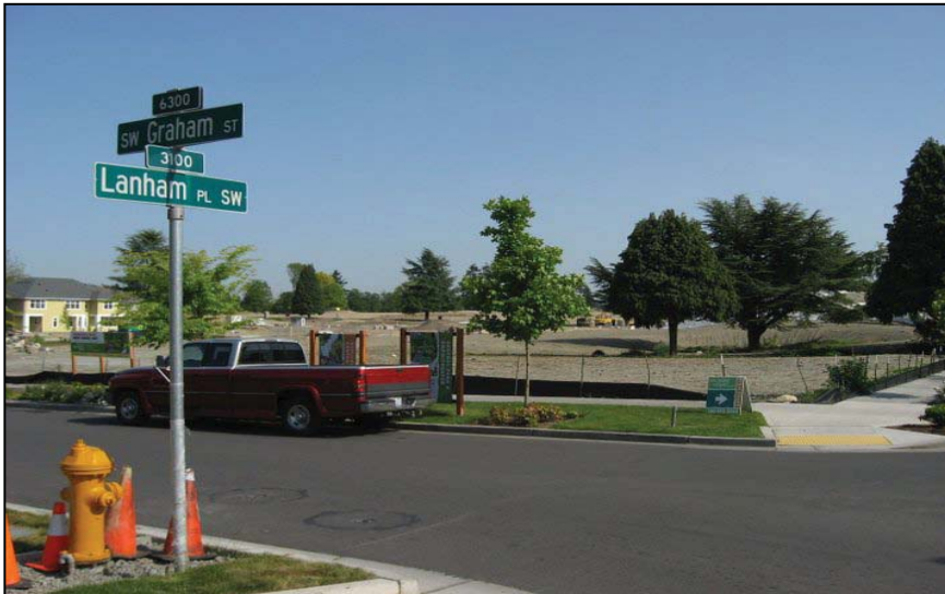
Tree Preservation during construction, Seattle, WA (USEPA, picasaweb)
