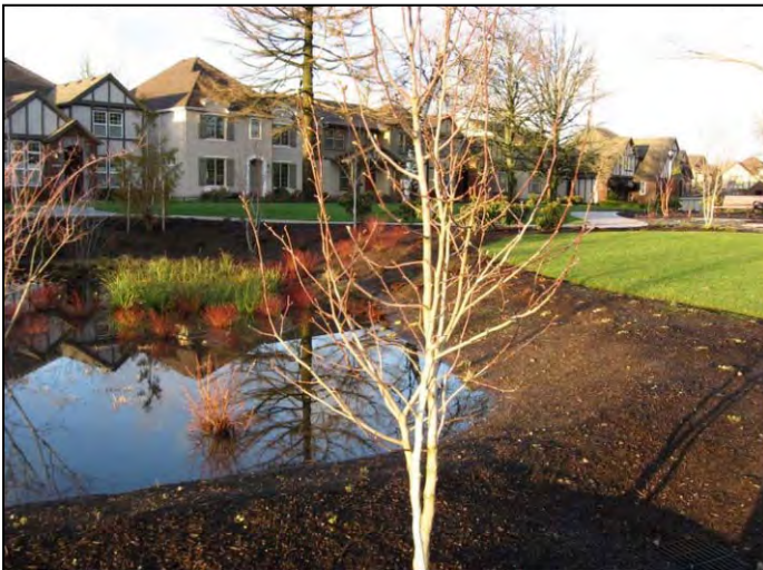
Pond collecting runoff from rooftops, sidewalks, and yards, Wilsonville, Oregon (USEPA,
