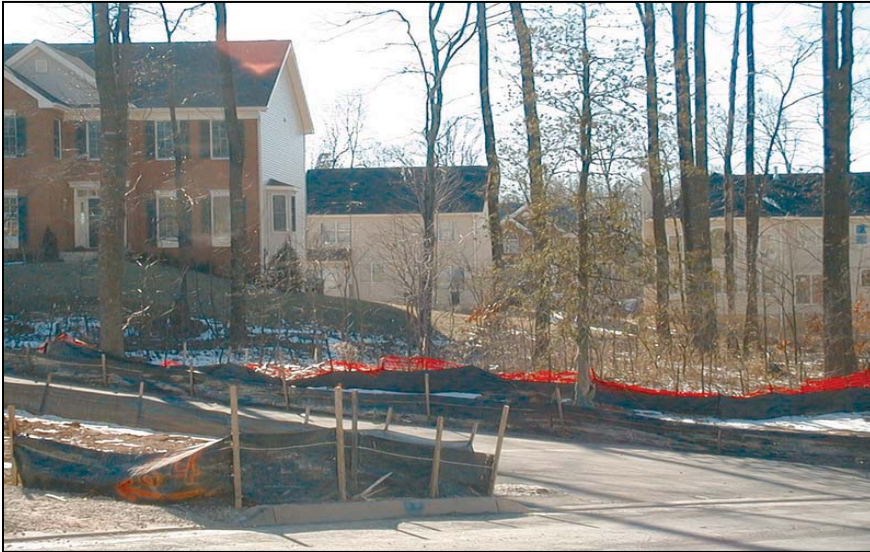
Undisturbed areas are protected during construction (Lake County, OH Stormwater Management Department)
