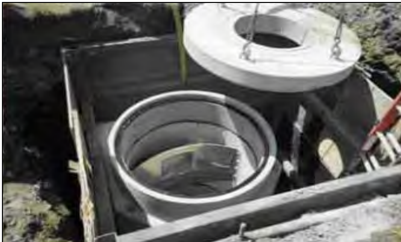
Installation of hydrodynamic separator (Johnson County, Kansas Stormwater Management Program)
